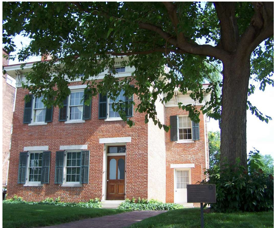
Quincy Underground Railroad Museum: Dr. Richard Eells House
